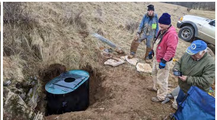
The installed gate
