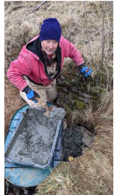
Rick shoveling quickcrete
